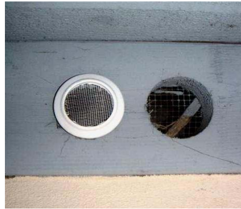
Figure 2d, Soda Can Under-eave Vent Insert (Cost is approximately 10 cents each - cost of soda can redemption value or $21.00/ 2000 sq. ft. home)
