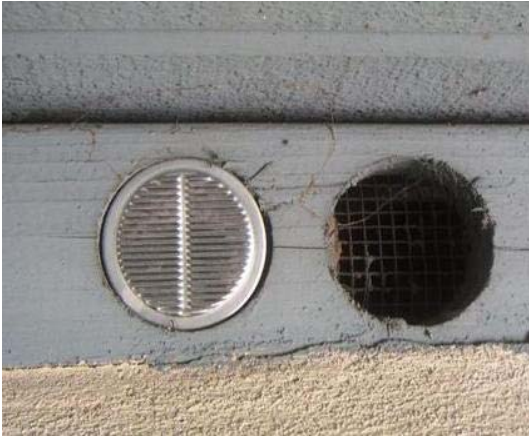
Figure 2c, Louvered Face Under-eave Vent Insert (Cost is approximately $3.00 each or $210 / 2000 sq. ft. home)
